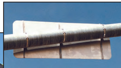
Mast Arm Sign Installation
